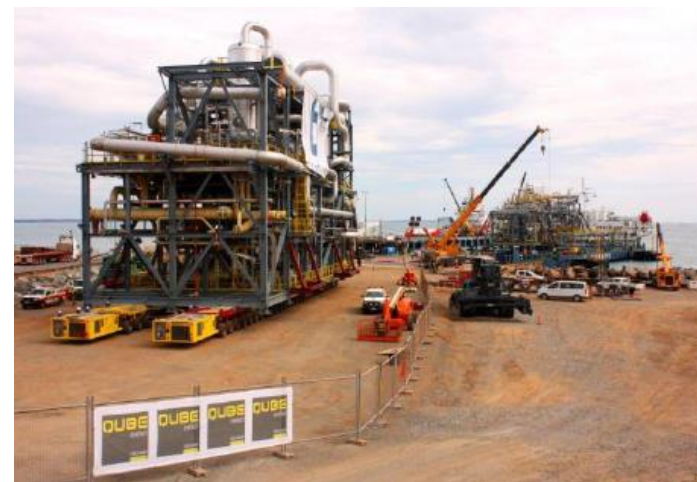
Handling of Yara Pilbara ammonia plant module, Dampier, WA Source: Qube
